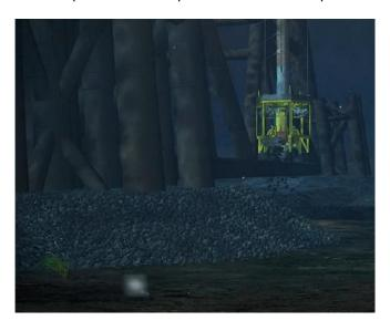
Fig 2 – Example of rock being placed via fall pipe end and ROV
